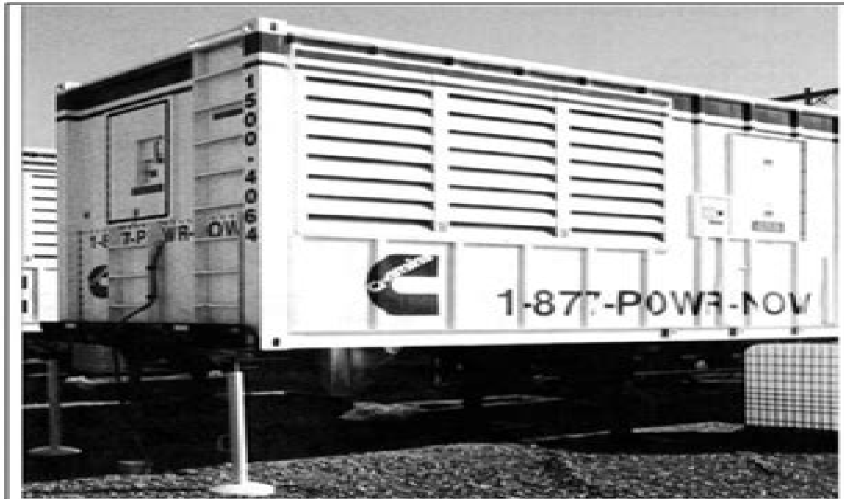
Jack Stands at Nose of Container
