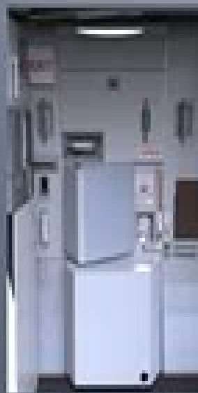
TYPE I DOOR EMERGENCY EXIT
